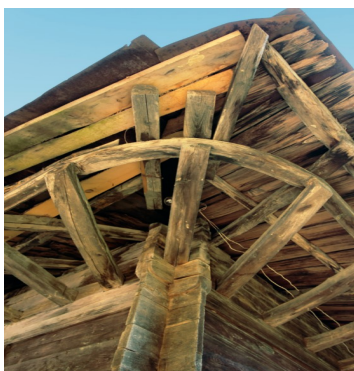
6. Village Takidzebi. Roof construction of a residential house.
