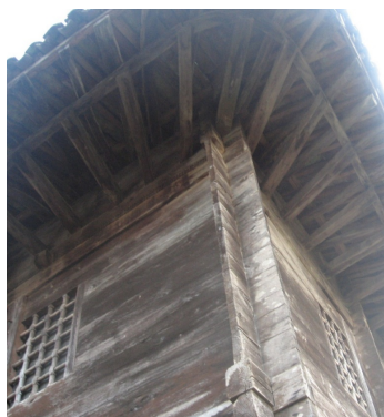
5. Kvirike. Mosque roof construction.
